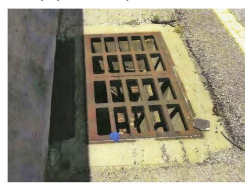
The trial court awarded Perkins \$93,362.97 in actual damages. In its order, the trial court found the overflow gap as installed was much wider than the gaps in the grate itself and presented a foreseeable hazard to the traveling public, which SCDOT failed to remedy. The trial court concluded SCDOT was liable for Perkins' injuries, and Perkins was not negligent in leaving her stalled car and attempting to cross the road to safety under the circumstances.
